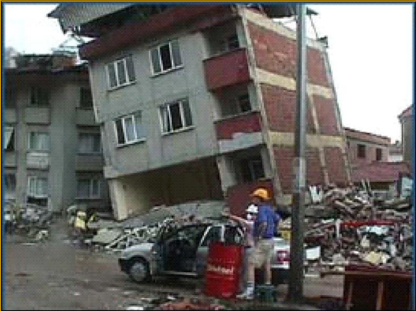
Foundation failure caused by liquefaction damaged this apartment building. Photo: USGS/Ft. Collins, CO
