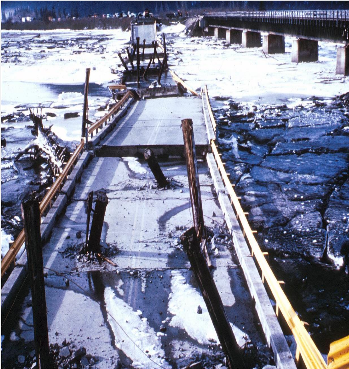
Bridge & Rail System Suffer Displacement
