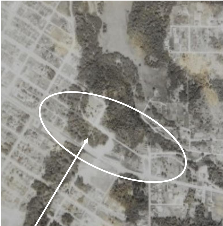
Earlier Photo shows the amount of fill over White Creek Area
