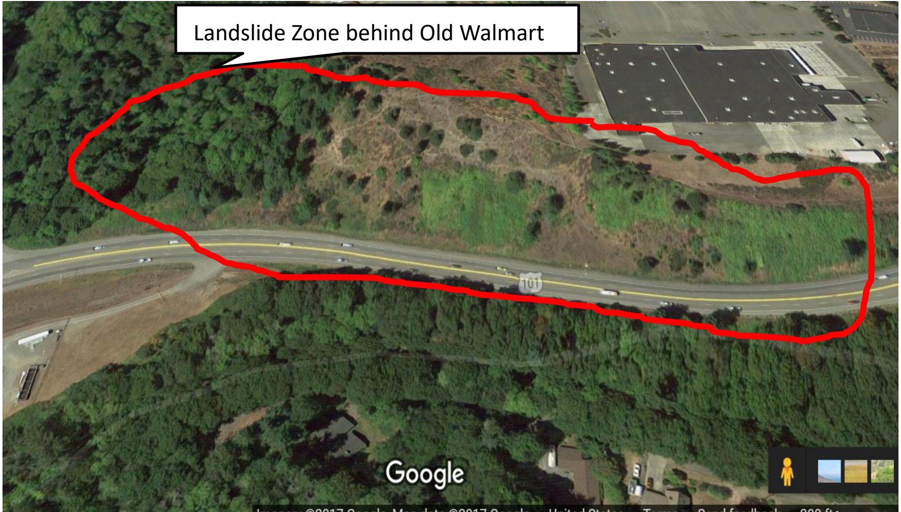
HIGHWAY 101 MORSE CREEK LANDSLIDE ZONE
