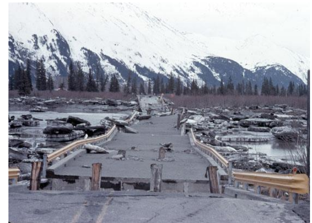
Bridge & Rail System Suffer Displacement
