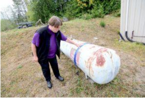
Donna Buck shows how the Joyce Emergency Planning and Preparation group wants residents to secure propane tanks, which would reduce the risk of fire in the event of a catastrophic earthquake. (Jesse Major/Peninsula Daily News)
