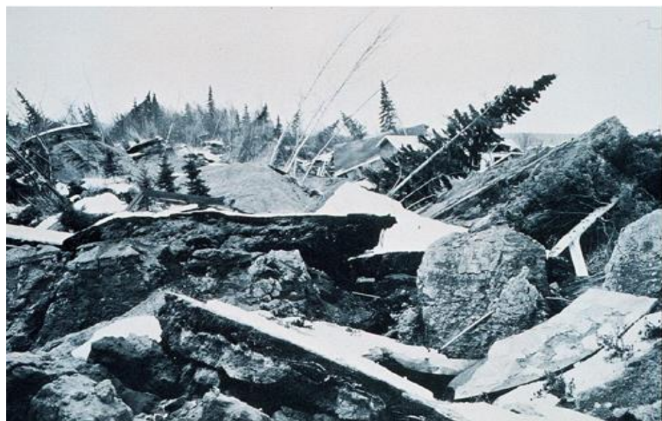
Earthquake damage at Turnagain, Anchorage, Alaska 1964
